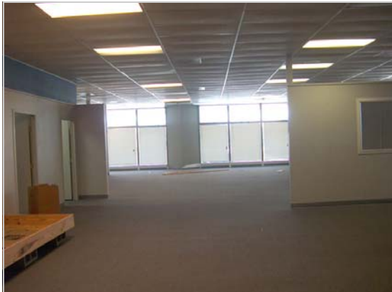
View of Offices and Large Work Area from Back of Space
